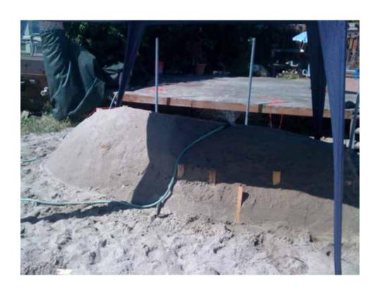
Having reached the top of the stakes the sand pile is ready to be formed
