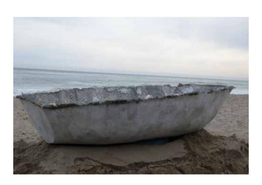
can now be removed and the inside finished with more mortar.
