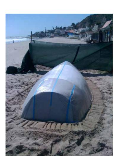
The first layers of chicken wire which will reinforce the concrete hull can now
