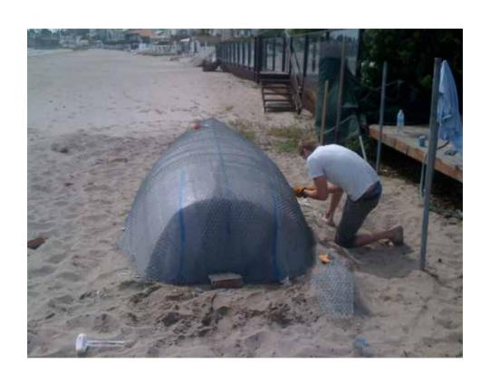
The layers of chicken wire are held together with wire to make a single tight layer of mesh about 3/4-inch thick.
