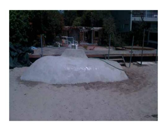
The sand is dug out from under the shell of the hull.
